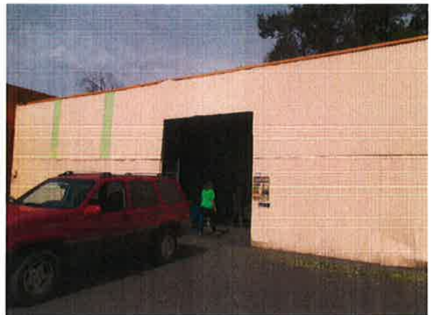
Photo 6 South section of metal building looking north.
