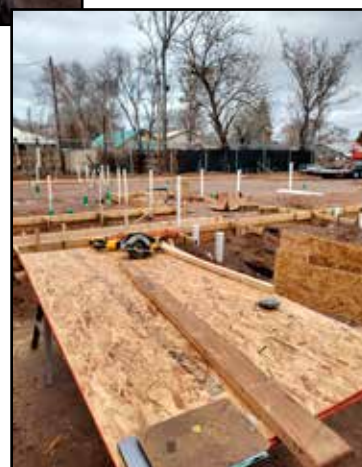
Plumbing stub outs on the new building site
