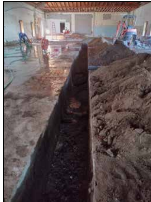
The pictures show the work beginning on the interior of the main building. Trenches being dug for water and sewer lines.
