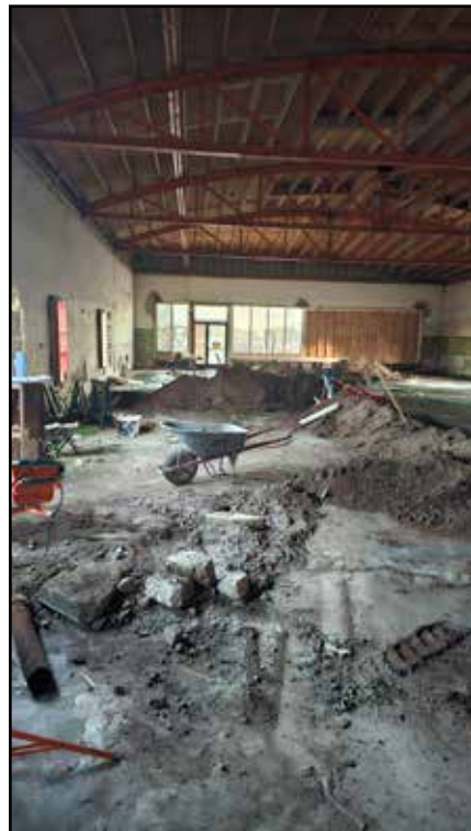
The pictures show the work beginning on the interior of the main building. Trenches being dug for water and sewer lines.
