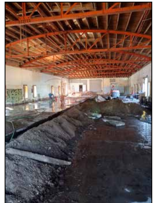
The pictures show the work beginning on the interior of the main building. Trenches being dug for water and sewer lines.
